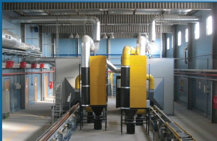
Rough grinding station ПГШ-01
